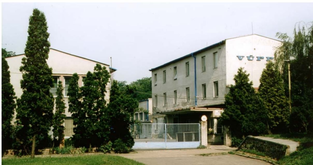
The second complex, the Development Base of Food-Processing Machinery, which is located in Hrušovany nad Jevišovkou
